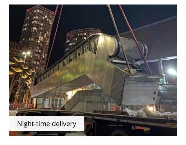
Fortunately, there was no major or significant building work needed, and once in progress, the removal and installation of the four escalators only took two weeks to complete. Fixings, assembly, making good, testing and commissioning were all undertaken during the daytime and behind hoardings.
